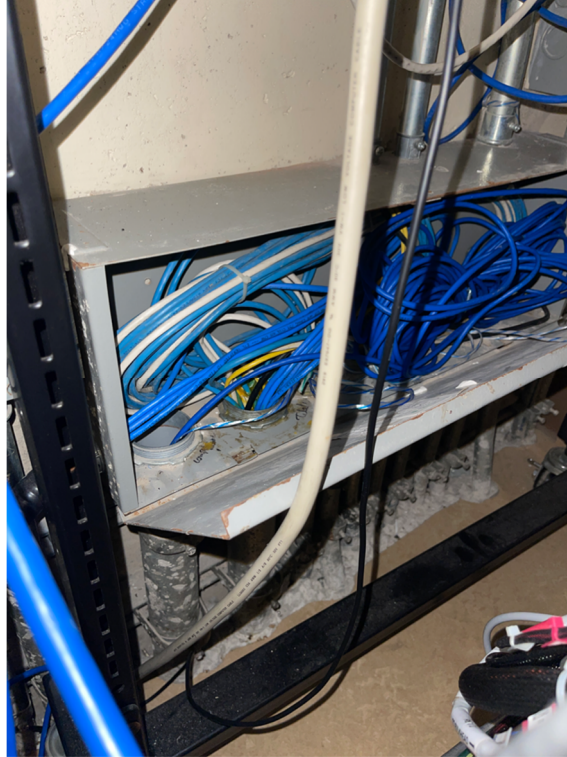
Photo 3.3.1-3: Existing Data Cable Junction Box Inside Closet of Control Area 1F222
